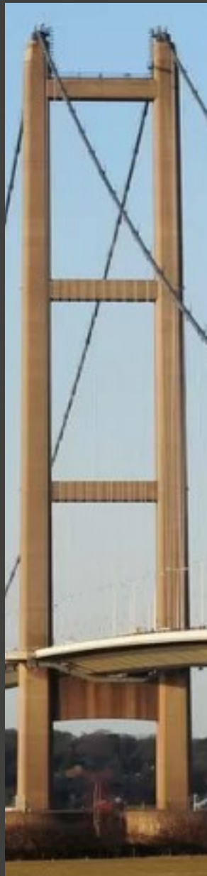
The Humber Bridge,, opened in 1981 by HM Queen Elizabeth II. It held the world record for the longest single span until 1998.
